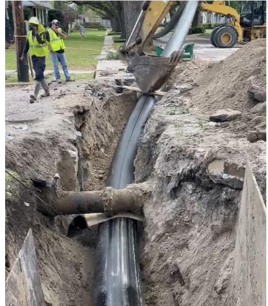
Force main installation taking place on Memphis Street in Lakeview.
