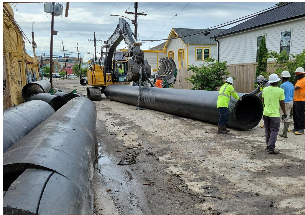
JIRR Work | Transmission Main Replacement on Eden Street
