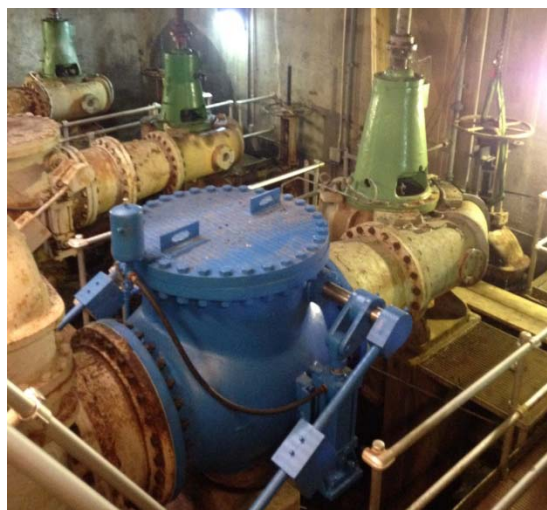
Effluent Pump 2 Check Valve Replacement System
