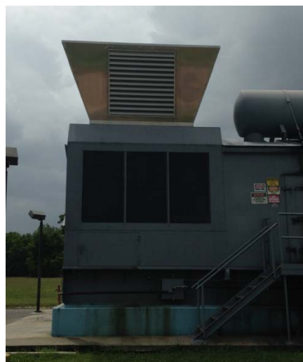
Emergency Generator Intake Air Filtration
