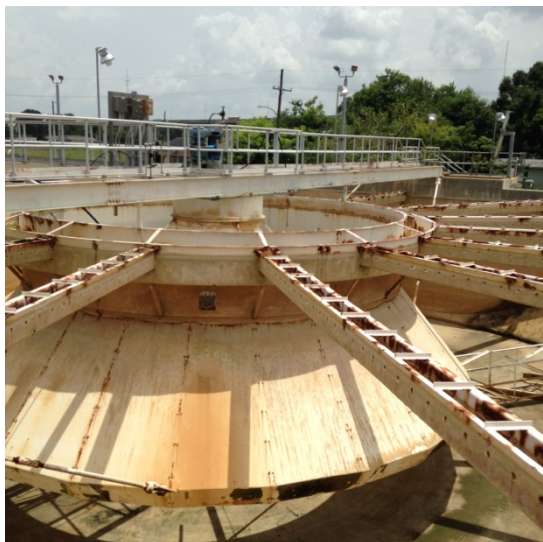
Corrosion on Clarifier
