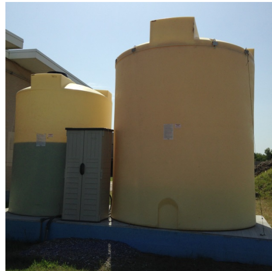
New Hydrogen Peroxide Odor Control System
