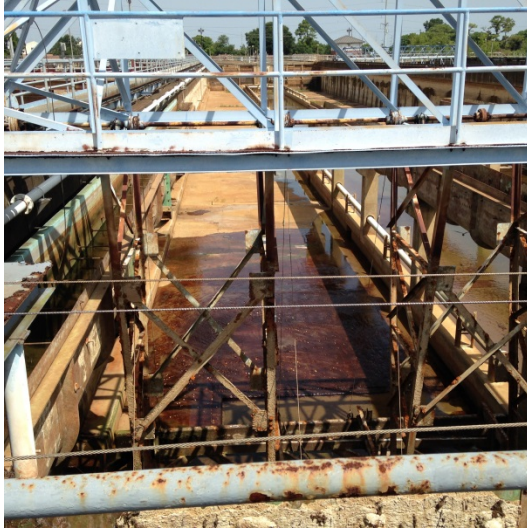
Sedimentation Basin Down for Repair
