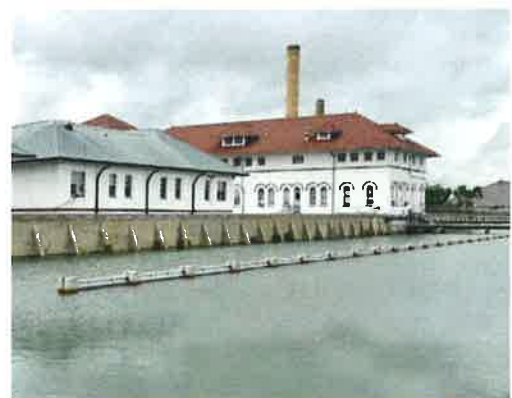
Carrollton Water Purification Plant
