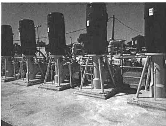
New Recycle Pumps in Service
