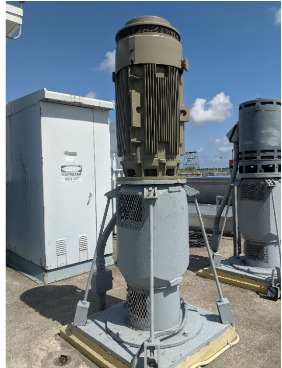
New High Efficiency Motor on RAS Pump
