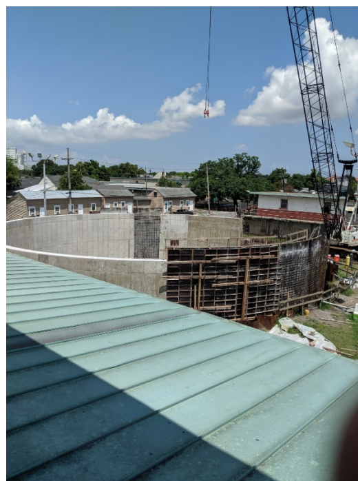
Clarifier 1 under construction
