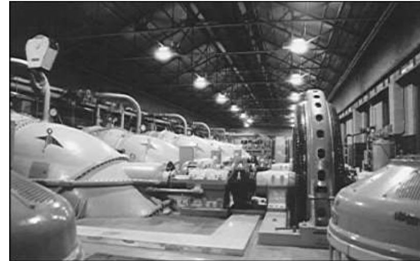
Figure 60. Drainage Pumping Station No. 6. View of interior looking east; in the foreground are 250 cfs vertical centrifugal pump motors. The remainder of the pumps are Wood screw pumps; in the foreground are two 12" pumps, and in the background are four 14" pumps.
