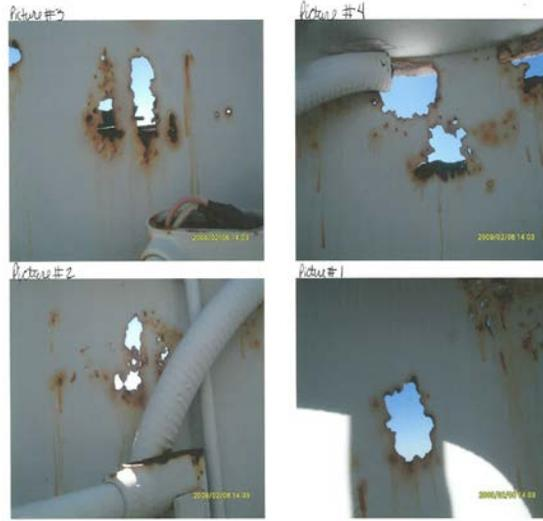
**Figure 5-15: 2009 Inspection Photos of Elevated Storage Tank**
