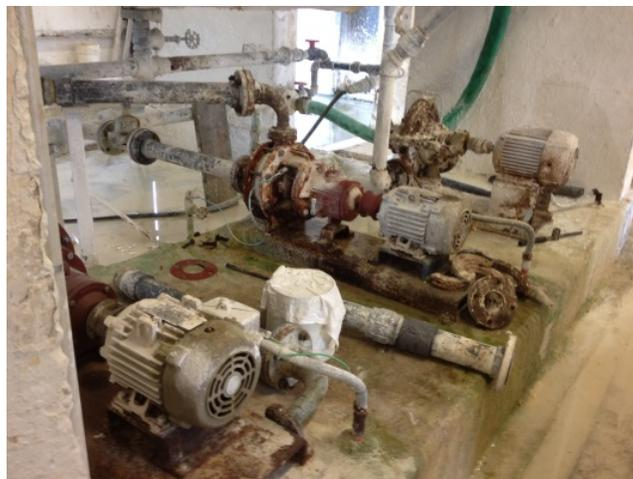
**Figure 3-40: Lime Feed Pumps**
