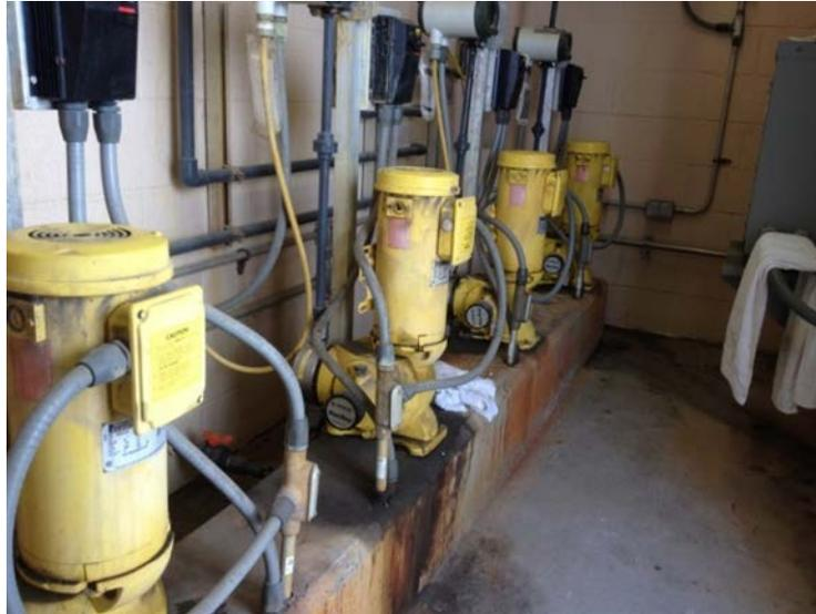
**Figure 3-58: Polymer Feed Pumps**
