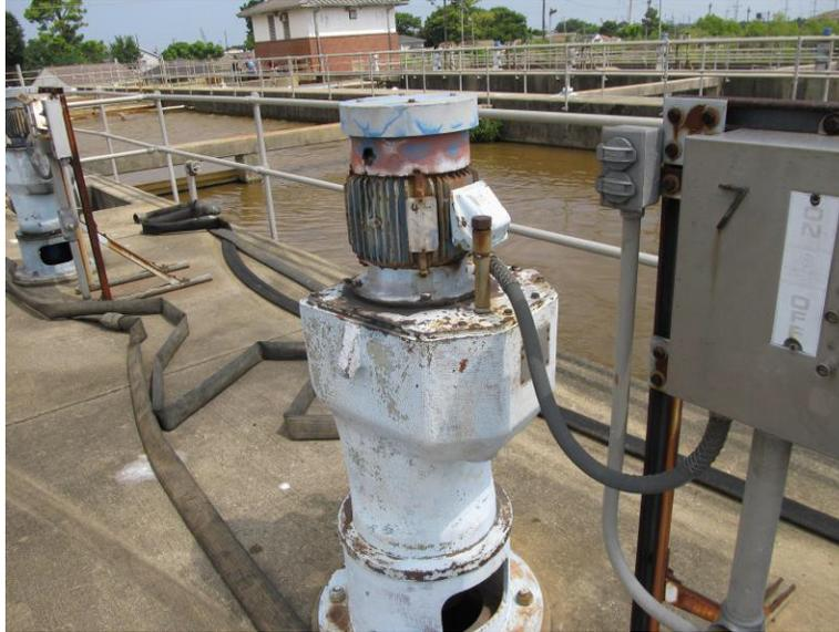
**Figure 3-7: L Basin Paddle Driver at Deck Level**
