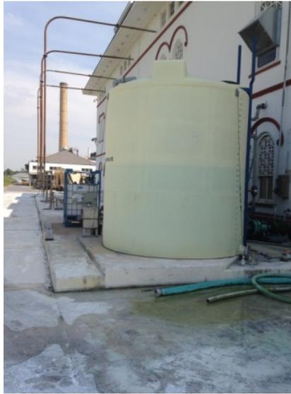
**Figure 3-55: Polyphosphate Storage Tank**
