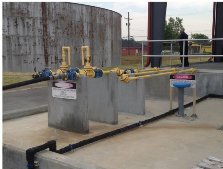
**Figure 3-28: NaOCl Unloading Piping**
