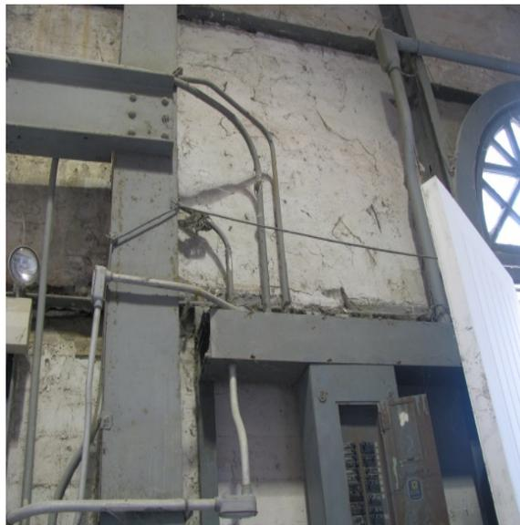
**Figure 4-4: Deteriorated Electrical Equipment**
