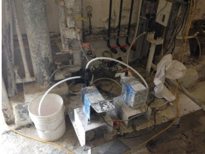
**Figure 3-56: Polyphosphate Feed Pumps**
