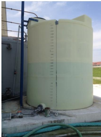
Figure 3-54: Polyphosphate Storage Tank
