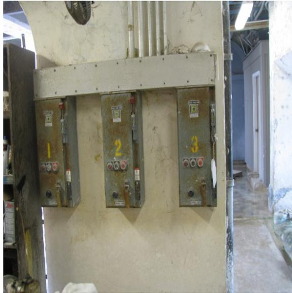
**Figure 4-6: Deteriorated Motor Starters**
