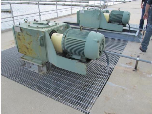
**Figure 3-11: Flash Mixers (with redesigned base-back mixer)**
