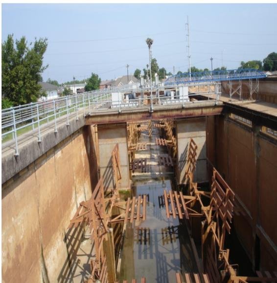
**Figure 5-1: Dewatered G3 Basin with Flocculators**
