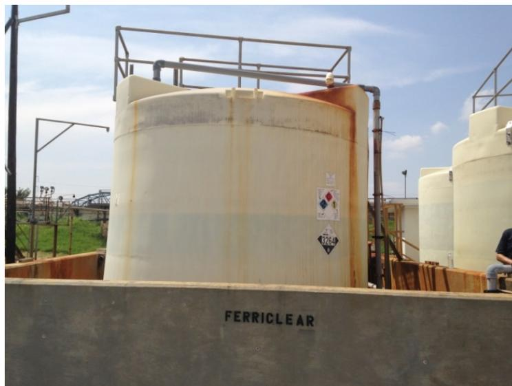
**Figure 3-42: Ferric Sulfate Storage**
