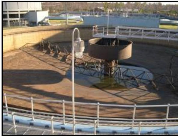
**Figure 30. Jammed Rake in Primary Clarifier**
