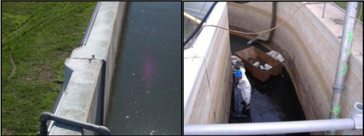
**Figure 17. Wall Separation in Effluent Channel**
