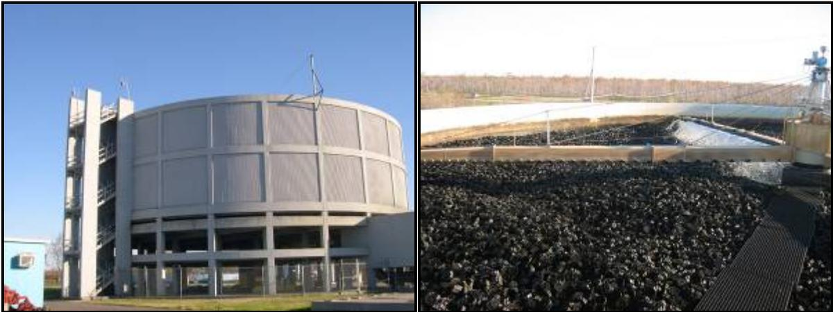
**Figure 29. Trickling Filter & Packing Media**
