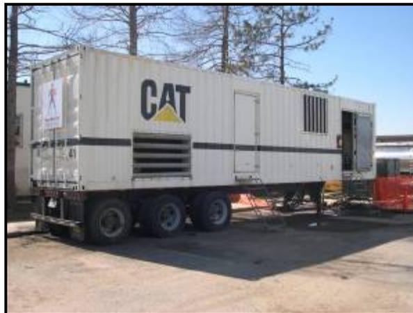
**Figure 22. 1.5 MW Generator On-site**
