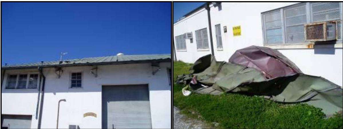
**Figure 36. Roof Damage to Maintenance Building**
