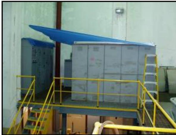
**Figure 10. Relocated Turbine No. 5 Switch Gear**
