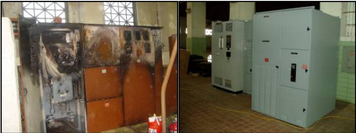
**Figure 9. Damaged/New Turbine No. 3 Switch Gear**
