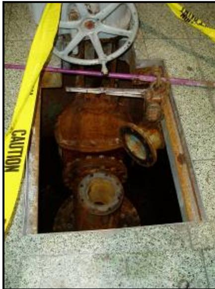
**Figure 14. Corroded Elbow - Pump No. 4**
