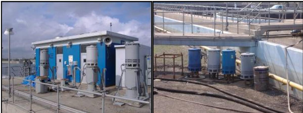
**Figure 20. Solids Transfer Pumps**
