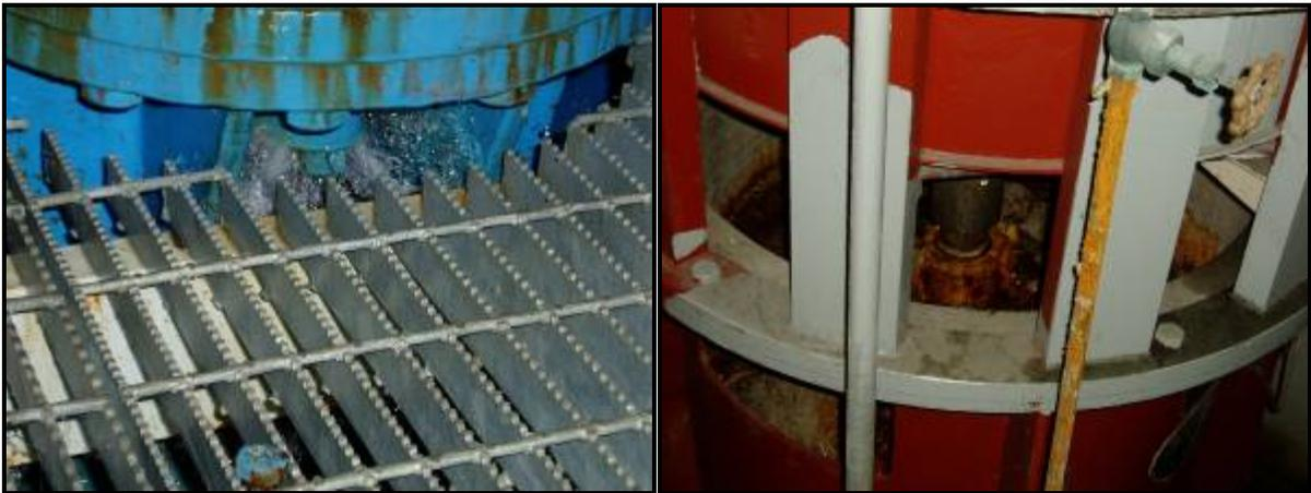
**Figure 15. Water Leaks – Panola & Claiborne Pumping Stations**
