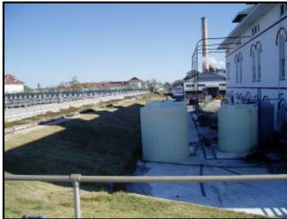
**Figure 37. Temporary Sodium Hypochlorite System**
