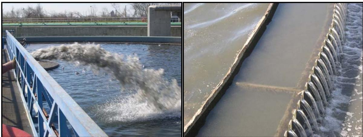
**Figure 24. Final Clarifier Being Drained & Final Clarifier Discharge**
