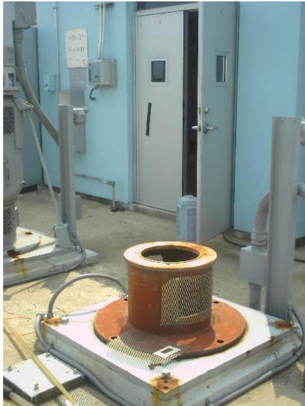
**Figure 8. RAS Pump Out for Repair**
