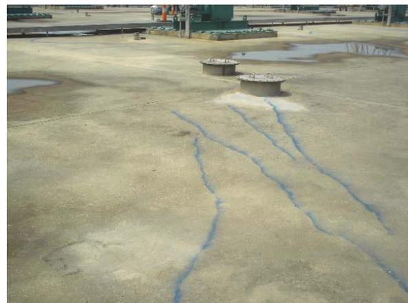
**Figure 7. Cracks in Deck**
