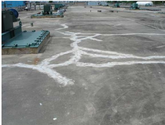
**Figure 7. Repaired Cracks in Deck**
