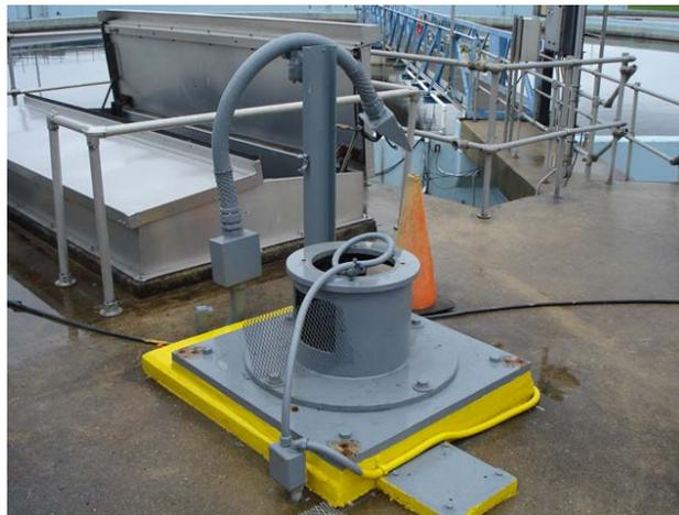
**Figure 6. RAS Pump Out for Repair**
