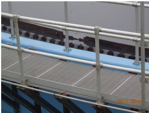
**Corrosion of Primary Clarifier Weir**
