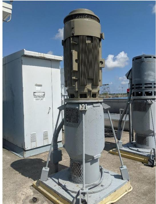
**New High Efficiency Motor on RAS Pump**
