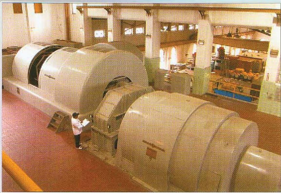
The S&WB operates its own electrical generating plant to produce power to run the massive network of drainage pumping stations. Underground feeders distribute power as needed during rainstorms.
