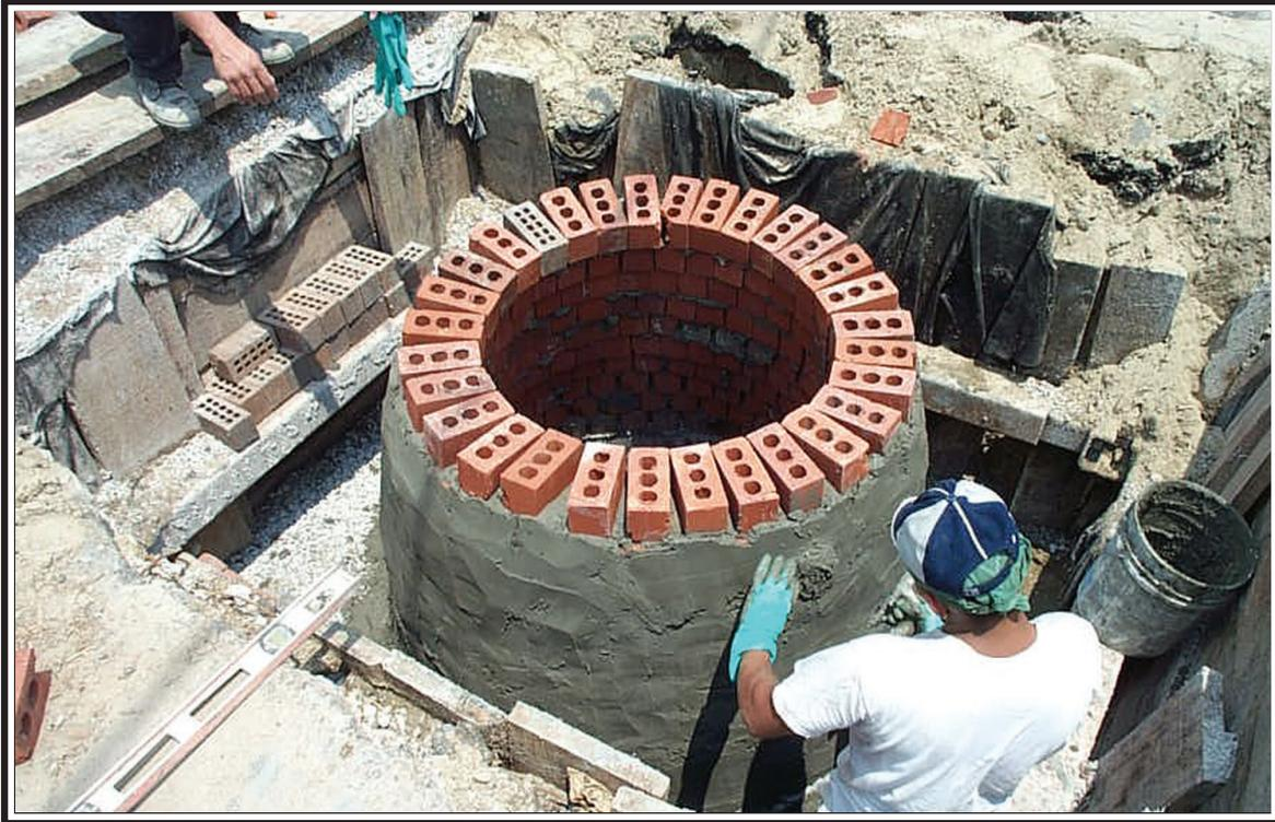
A major element of the Board's Sewer System Evaluation and Rehabilitation Program (SSERP) is the replacement of damaged, leaking or sinking manholes. Since 1998, approximately 4,800 sewer manholes have been repaired or replaced. Above, a manhole is under construction, and below, the completed structure is ready to be sealed into a new section of roadway.
