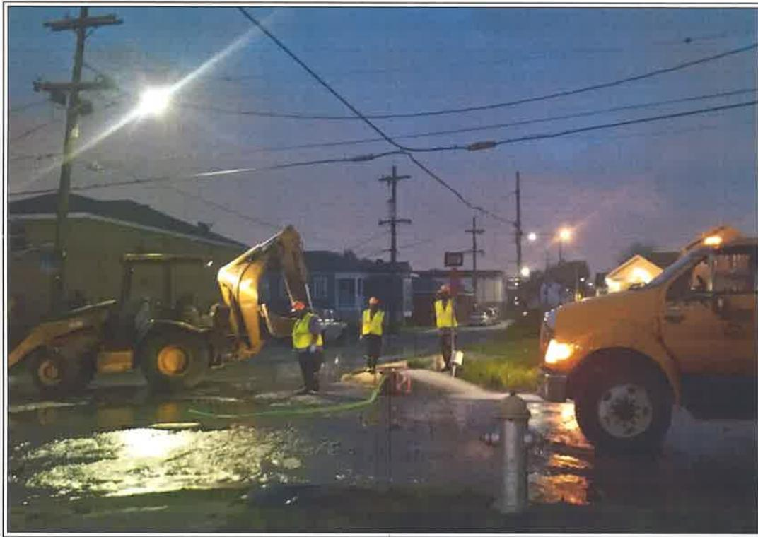
*Network crews work around the clock daily to deliver quality of life services of water, sewer and drainage to the residents of the city. A late night emergency water main break is shown being repaired.*
