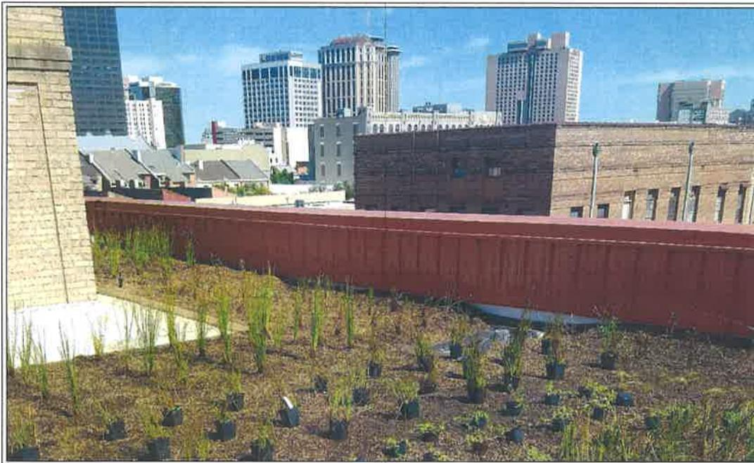
*Severage and Water Board's (S&WB) main office on St. Joseph Street has a new roof. It is a green or vegetated roof that will catch and hold rainwater to help reduce flooding and improve storm water quality. The roof will also provide additional insulation for the building and lower temperatures in the surrounding area. This project is part of the Green Infrastructure Program.*
