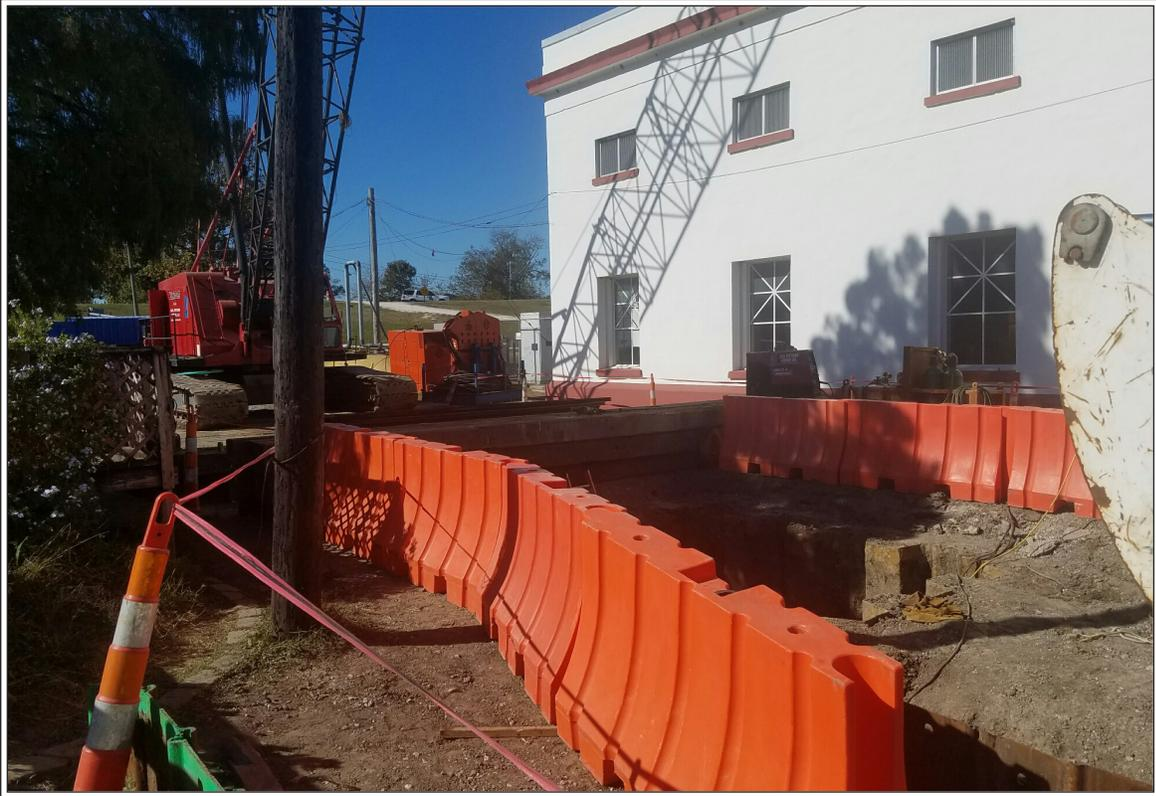
*The S&WB Onk Street Pumping Station Rehabilitation is part of the Hazard Mitigation Grant Program. The existing station has 4 pumps that pump water from the river to the S&WB Carrollton Water Plant to be treated. This construction will remove three pumps and replace them with brand new motors and pumps, along with new piping and auxiliaries. Completion is expected in 2019. However, high river levels can cause a delay in the construction outside the*
