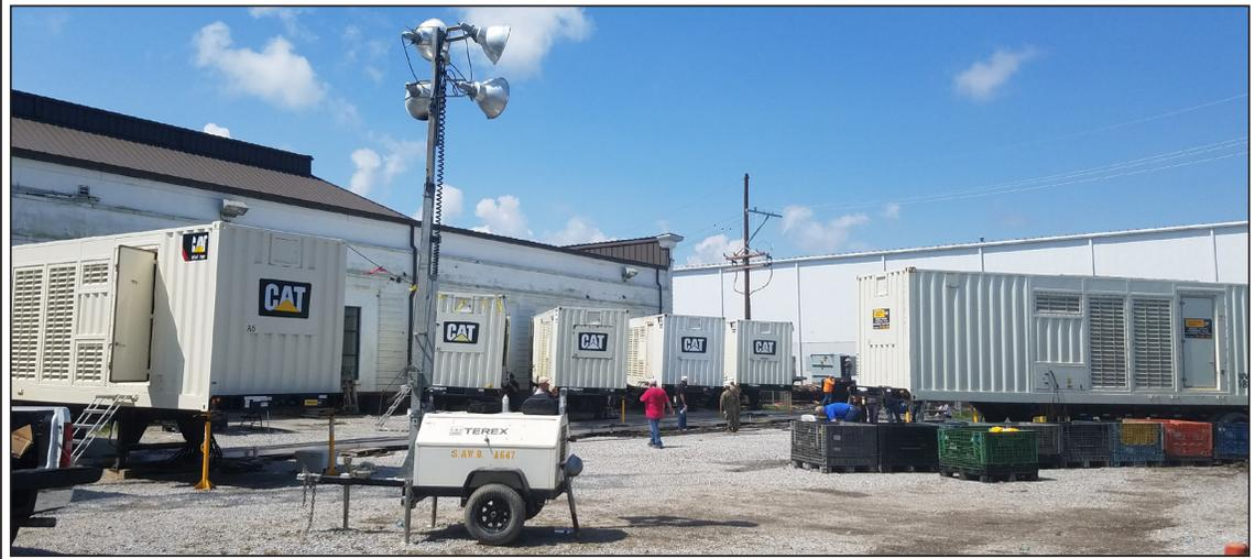
Generators were put in place at various facility sites to provide an uninterrupted power source to critical operations. They were designed to increase and insure reliability in the event of a commercial power interruption. Top generator photo: S&WB Carrollton Plant. Bottom generator photo: S&WB Central Yard
