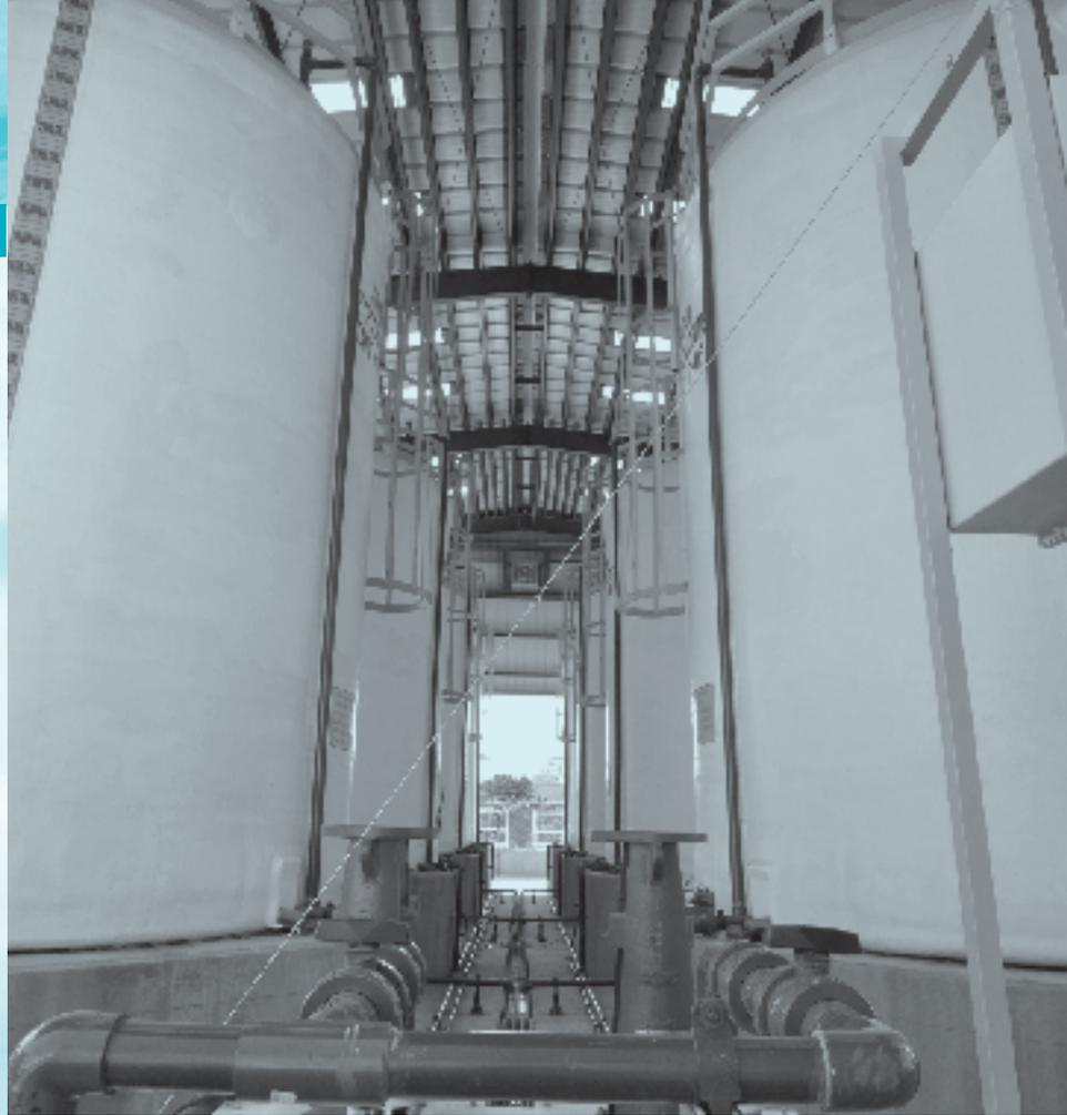
The Sewerage & Water Board's staff is constantly developing and exploring new processes to improve its operations. One such project is underway at the Carrollton Water Purification Plant. The Sodium Hypochlorite Bulk Storage/Feed Facility is set for completion in July of 2012. It will eliminate the need for transporting chlorine into the plant by rail and storing it on the plant grounds. Instead, the Board will use the safer sodium hypochlorite for disinfection in the purification process.
