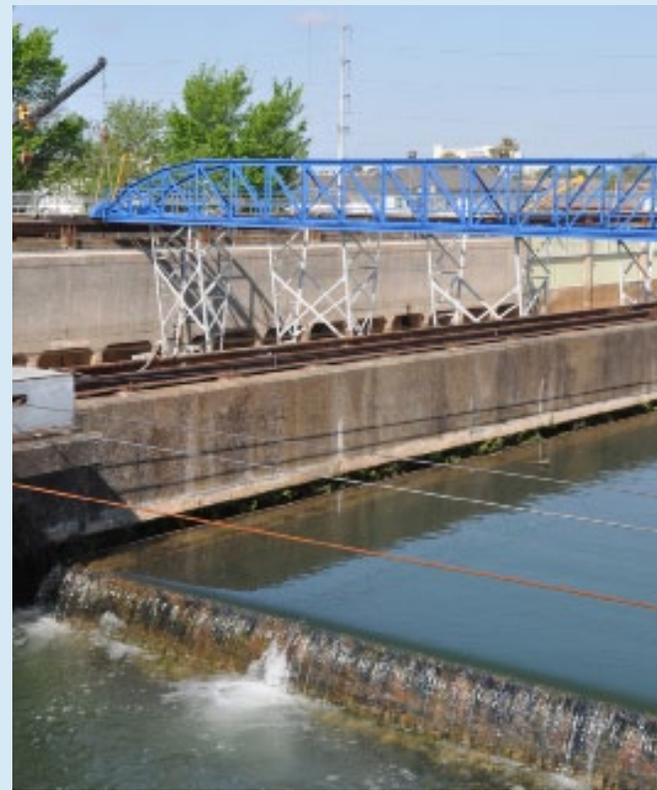
*The East Bank Water Treatment Water Plant has four basins in which water from the Mississippi is brought in and processed into quality potable water for the city of New Orleans. The basins must be removed from service, periodically, one at a time to perform cleaning and scheduled maintenance.*
