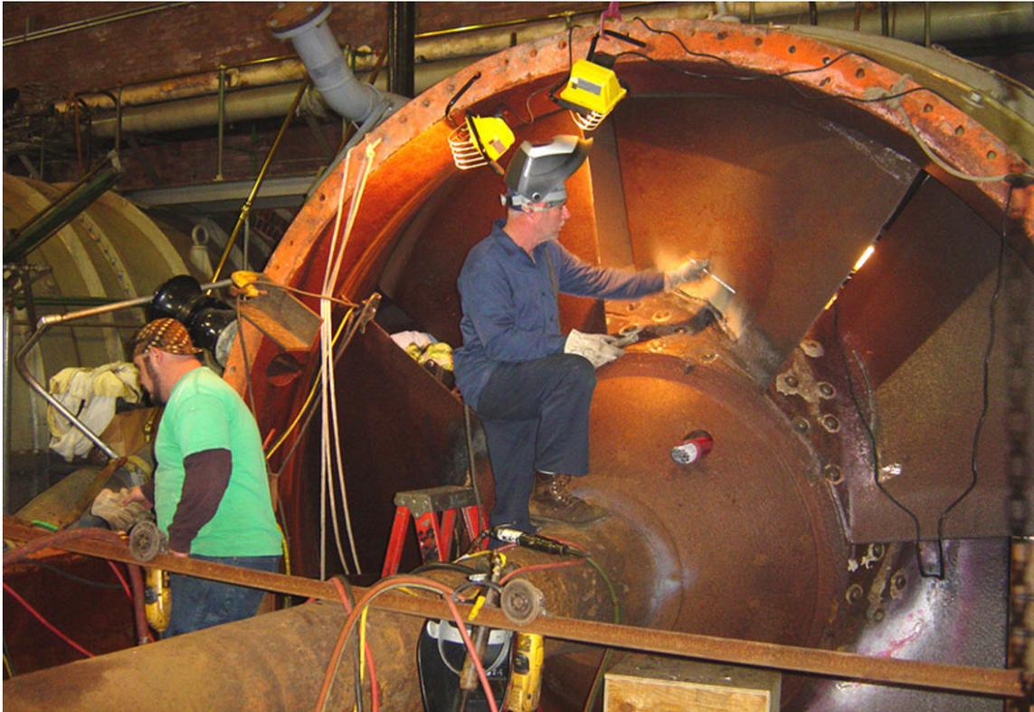
When one of the pumps at Drainage Pumping Station No. 3 began to “chatter” and make a loud noise, it was discovered that 5 of the 8 impeller blades were cracked. The Board’s own employees from Facility Maintenance disassembled the pump, gouged out the cracked areas and weld-repaired the blades.
