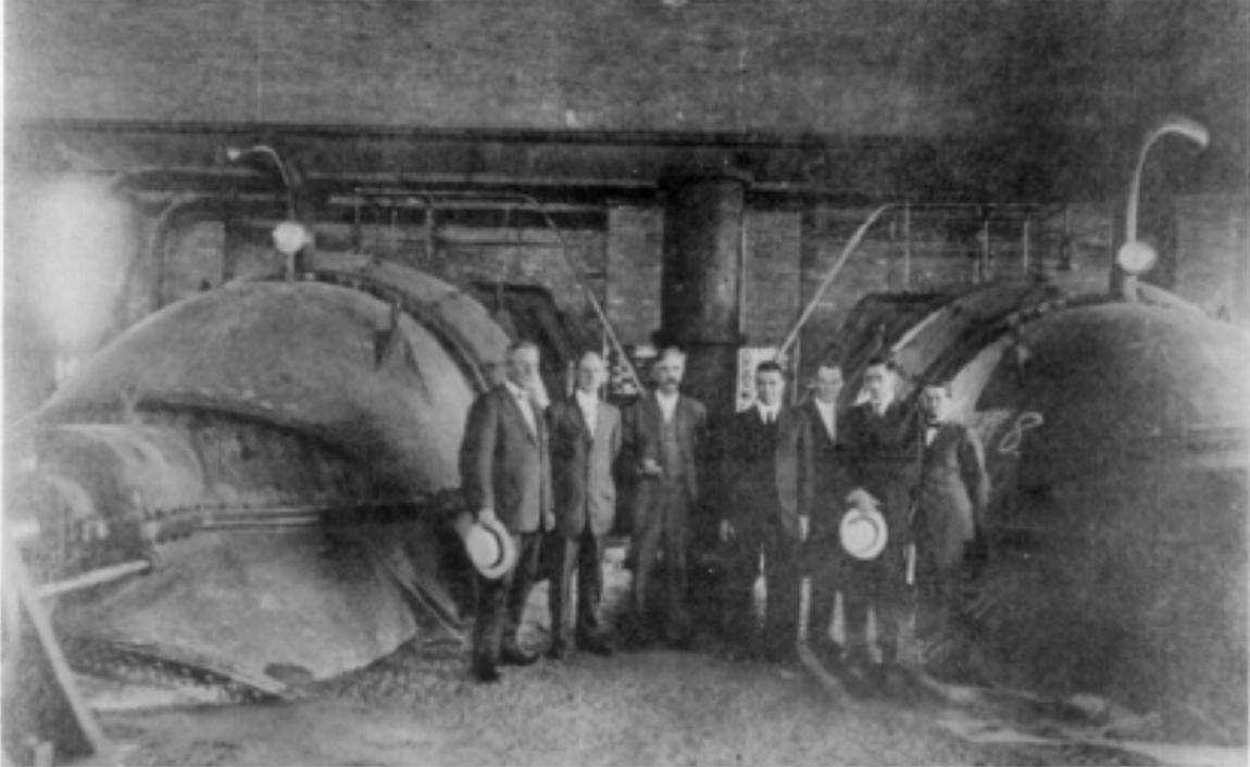
THEN - In 1915 the 12 ft Wood Screw Pump was the most advanced drainage pump in use. Wood's pumps were built all over the world after their successful operation in New Orleans was proven.
