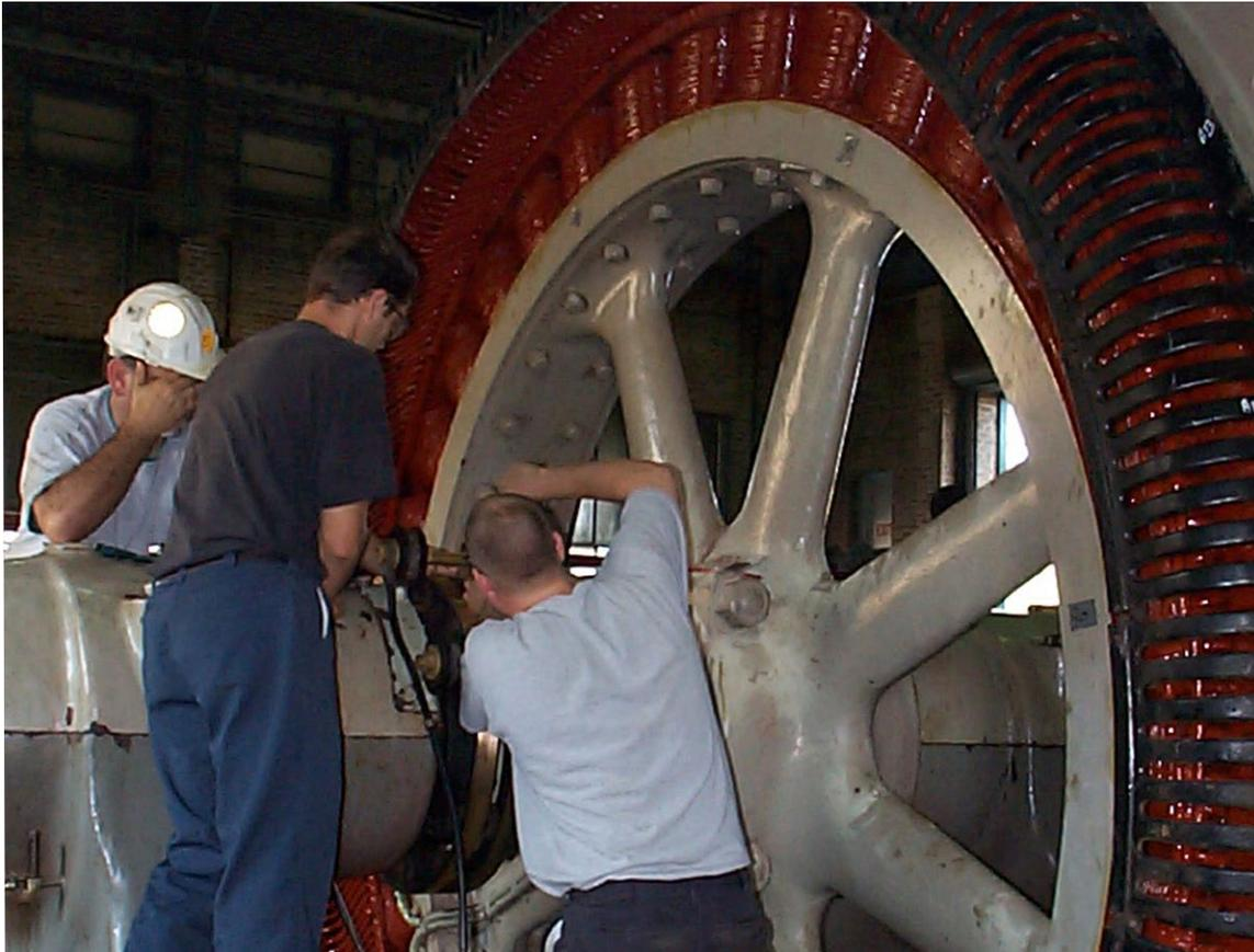
Flood waters from Hurricane Katrina submerged many of the giant motors which power the massive pumps of the S&WB's Drainage System. Within three days of the storm's passing, the Board had arranged for a team of experts from the General Electric Corporation to come to the City to work with S&WB staff to dry the motors and begin the re-winding process.
